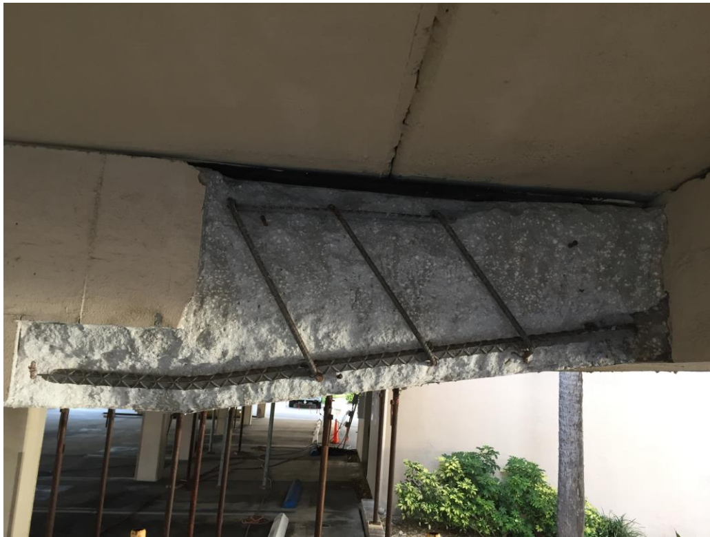
Picture 2: Concrete excavation
