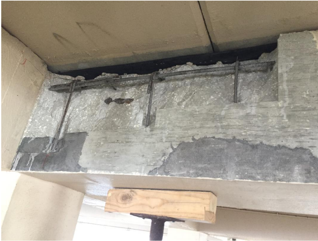
Picture 3: Concrete excavation
