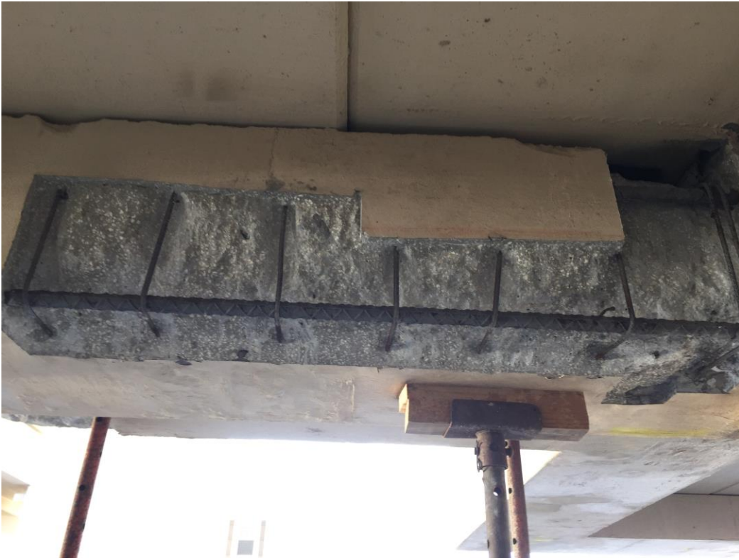
Picture 1: Typical concrete excavation
