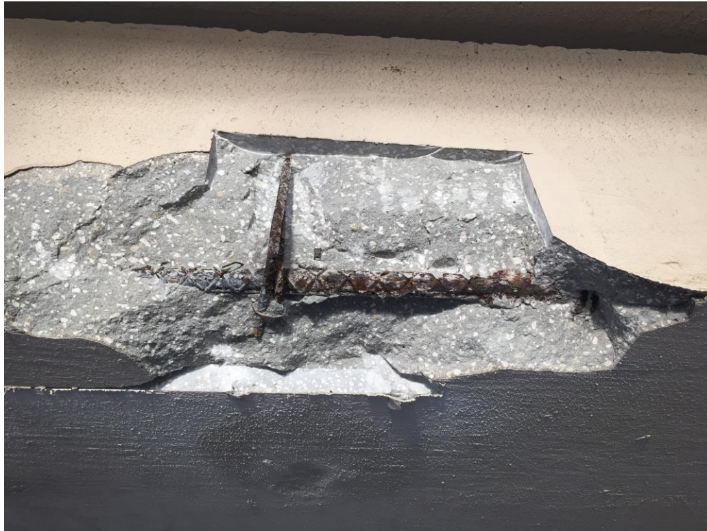
Picture 4: In-progress concrete repair
