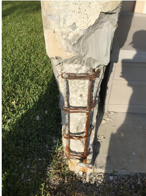
Picture 5: In-progress concrete repair
